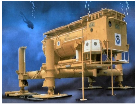
Owned by NOAA and managed by the University of North Carolina at Wilmington (UNCW), the AQUARIUS habitat is an 82-ton double-lock pressure vessel approximately 14 meters long by 4 meters in diameter. Photo: NOAA
